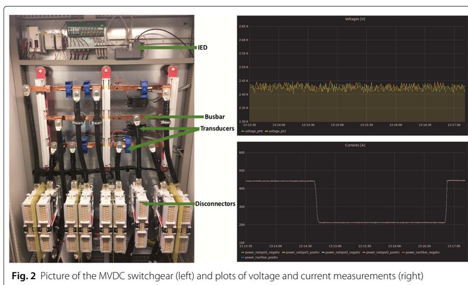
**Fig. 2** Picture of the MVDC switchgear (left) and plots of voltage and current measurements (right)
